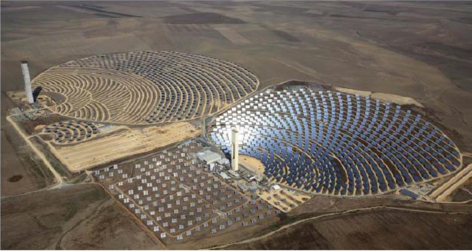
Figure 3-32: PS 10 central receiver solar tower facility near Sevilla, Spain (Abengoa Solar). In the background the PS20 facility can be seen under construction
