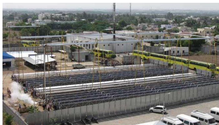
Fig. 5. Flat Mirrors with single axis tracking for power and water (flat mirrors –CSP KGSL-Coimbatore – single Axis tracking sun's movement)
