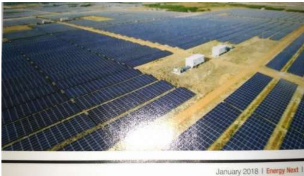
Fig.10 Mega watt or Utility scale Solar Power Plant System ( 100s MW )
