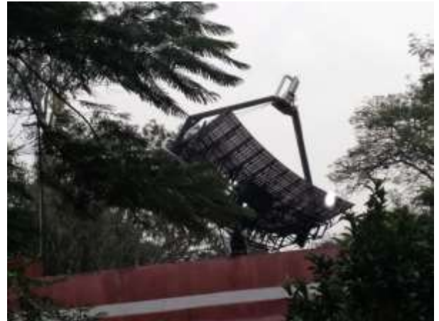
Fig.17 CSP* Concentrated Solar thermal for power generation (ABD,TNAU,CBE-Dual axis tracking installation)( ABD-TNAU coimbatore : Dual axis tracking of sun's movement
