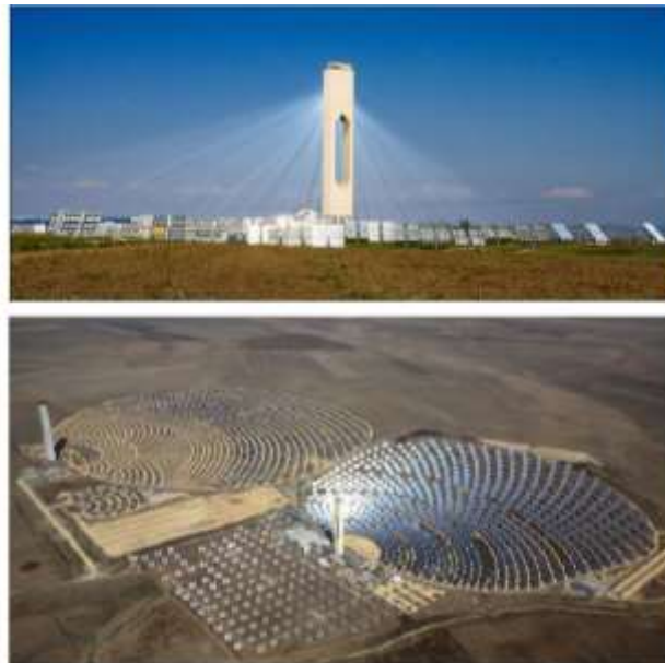
Figure 3-32: PS 10 central receiver solar tower facility near Sevilla, Spain (Abengoa Solar). In the background the PS20 facility can be seen under construction
