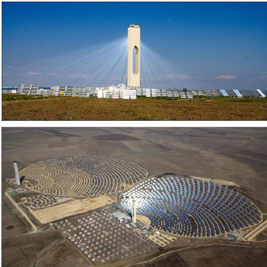
Figure 3-32: PS 10 central receiver solar tower facility near Sevilla, Spain (Abengoa Solar). In the background the PS20 facility can be seen under construction
