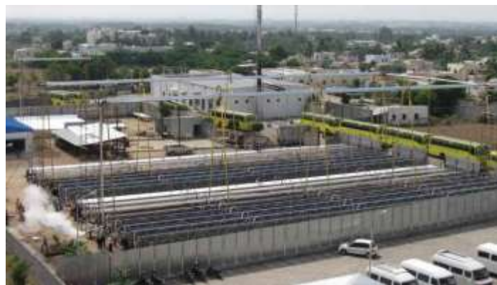
Fig.16 Flat Mirrors with single axis tracking for power and water (flat mirrors –CSP KGSL-Coimbatore – single Axis tracking sun’s movement)
